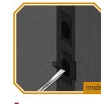
5 For Deadbolt and Latch **Strikeplates:** Chisel out holes for dustboxes. Chisel out cavity so deadbolt strikeplate and latch strikeplate fit flush with doorframe. For deadbolt strikeplate, cavity is \( \frac{1}{32} \)" deep For latch strikeplate, cavity is 3/32" deep.
