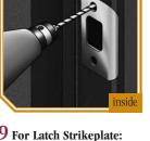
9 For Latch Strikeplate: Using latch strikeplate as a template, drill two 1/8" pilot holes
